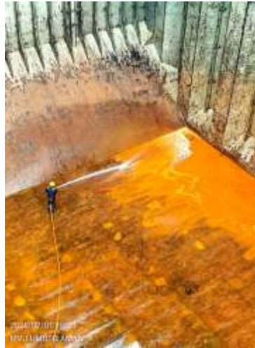
Gambar 2. Proses Cargo Hold Cleaning MV. Lumoso Aman.
