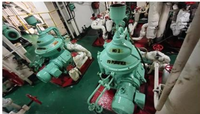
Gambar 3. Fuel Oil Purifier.
